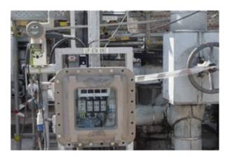
CMCP530 Velocity Monitors were selected to integrate the acceleration signal to velocity and provide the local OK, Alert and Danger Alarms along with the required 4-20 mA signal. CMCP505 Bright Red LED Displays were selected for easy operator viewing. A CMCP515 Universal Power Supply was provided to supply the +24 VDC required by the CMCP530 Series Monitors.
